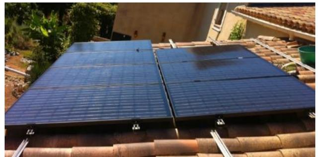
*Figure 7 : installation on K2 overlay system*
